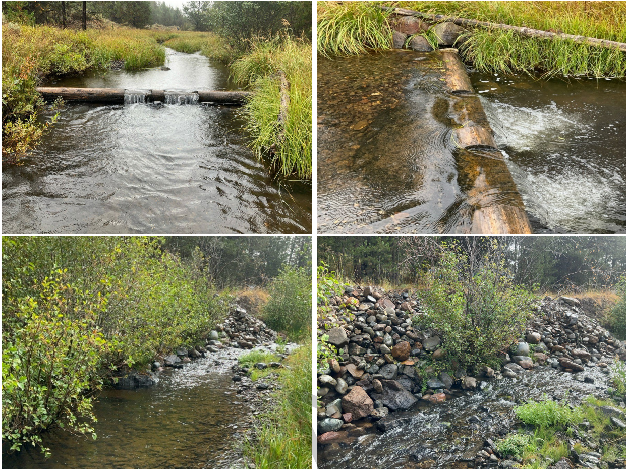
Figure 8. Images of placed wood and an armored bank located on Bull Run Creek.
